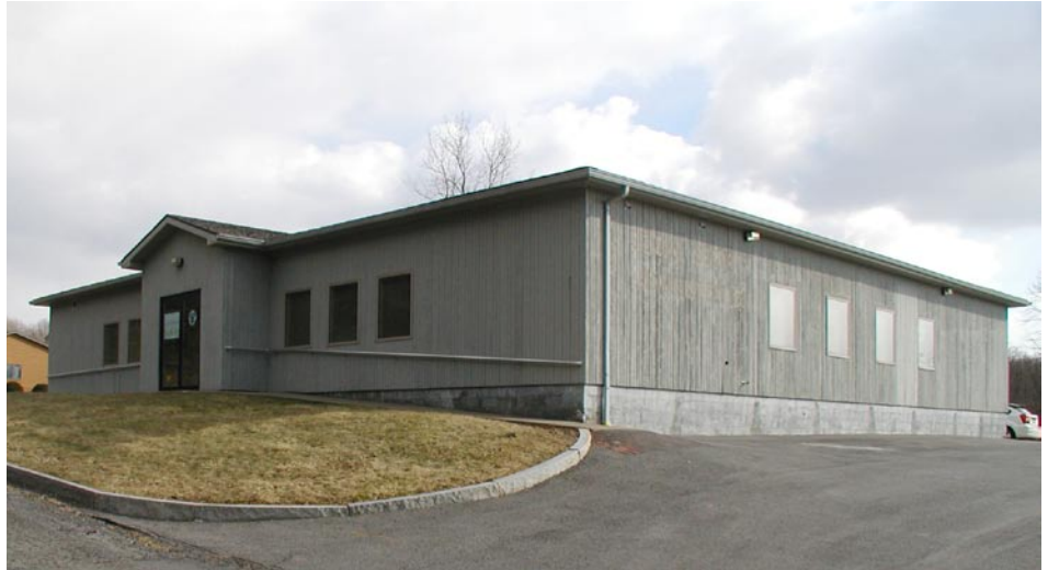
New quarters for Unity House's UES-Auburn, IPRT, and Independent Housing programs and services.
